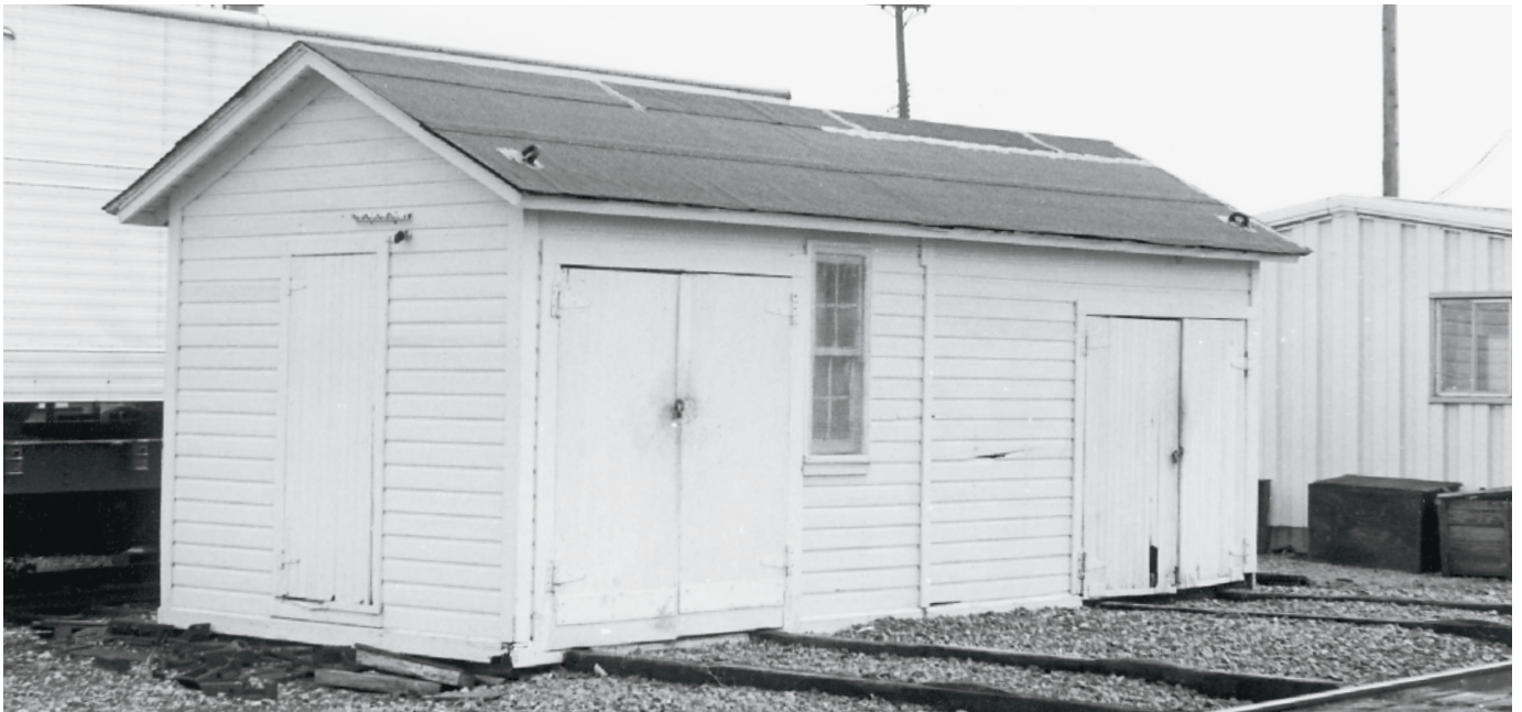
Two pairs of wooden beams leading to the track indicate that this old building is set up as a speeder shed. The well-worn walls show years of service; a seam down the middle indicates the structure was once half its current size.
