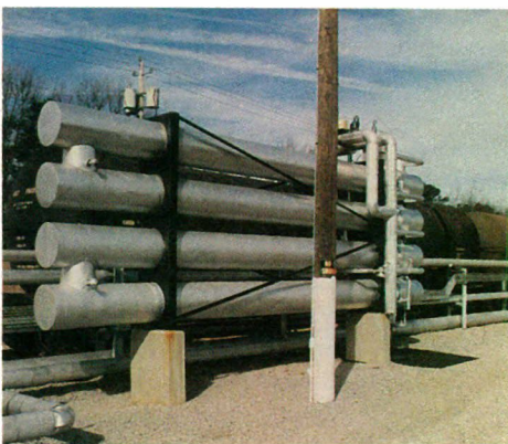
Fig. 7. PROTOTYPE HEAT EXCHANGER. This unit uses steam to heat the liquid asphalt so that it flows easily to a waiting tank truck.
