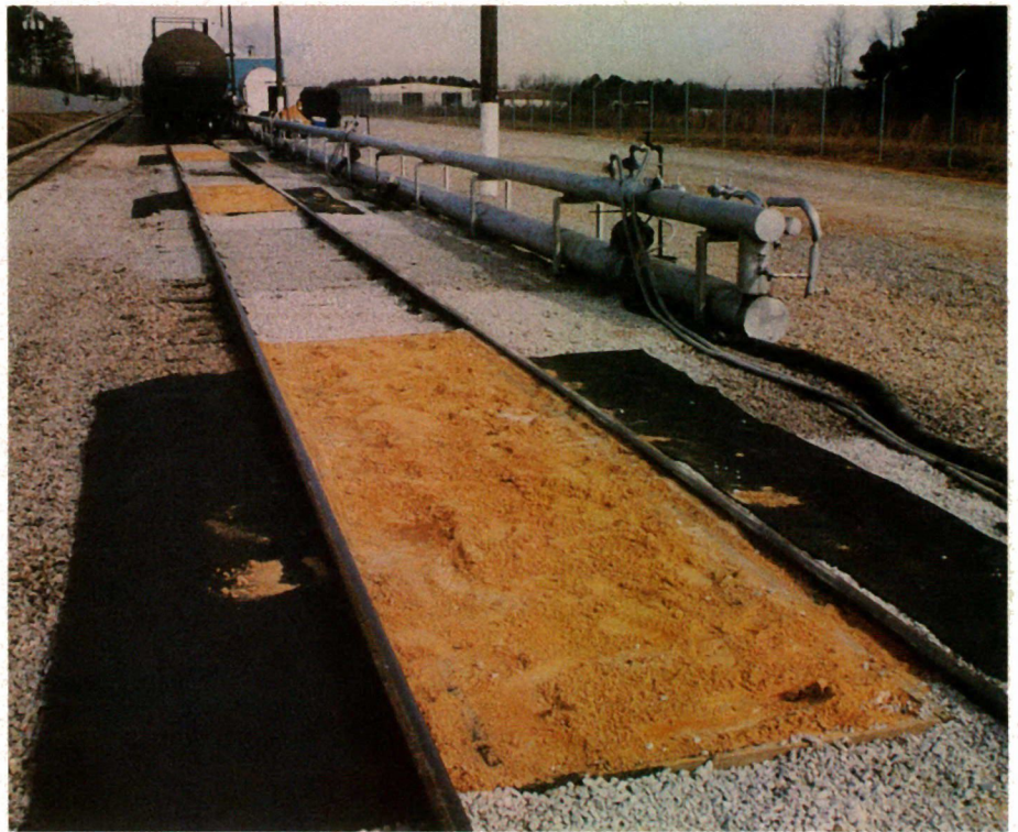
Fig. 13. TANK CAR UNLOADING AREAS. Sandboxes under each car catch spilled globs of asphalt.
