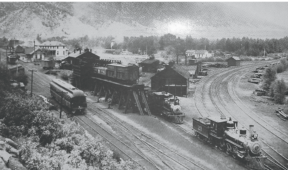
The yard at Basalt is sized for interesting operation but small enough to avoid overwhelming the layout. It's also a helper station. The main line runs off to the left while the Aspen branch curves to the right. David P. Morgan Library collection
