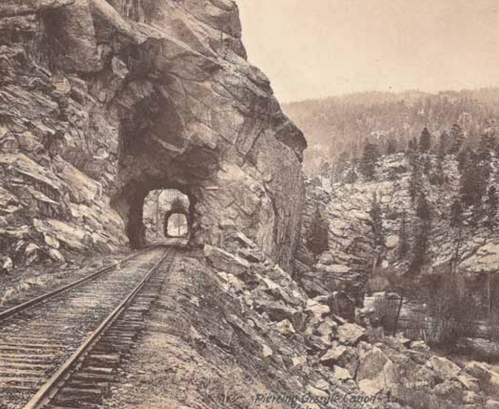
This photo of the tunnels bordering Granite Canyon documents the rugged terrain facing the builders of this pioneer Colorado standard-gauge railroad as well as the appeal of modeling these landmarks. Author's collection
