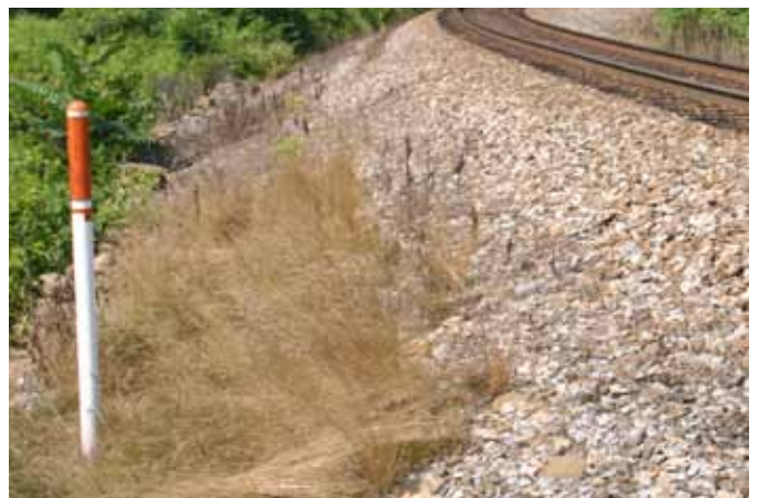
Today, fiber-optic cables are common along the right-of-way. Lineside markers like this one along the Norfolk Southern in Linden, Va., denote the buried cable's route.
