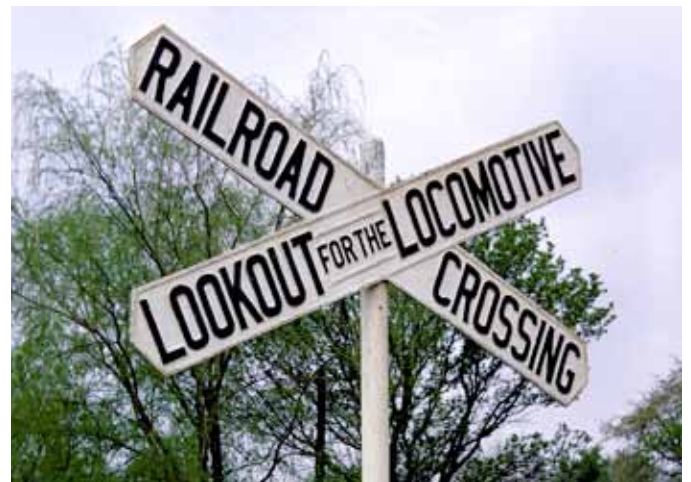
Although 90-degree crossbucks are now standard, these cast-iron crossbucks are at 50 degrees. This photo was taken in 1967 along the Pennsylvania RR in Denton, Mich.
