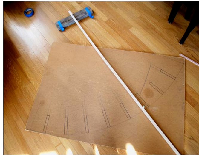
4. A template is made on a scrap using the dimensions already determined.
