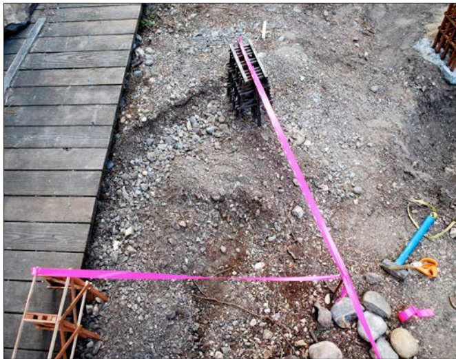
3. Using contractor's tape and a steel square to determine the center point of the curve.
