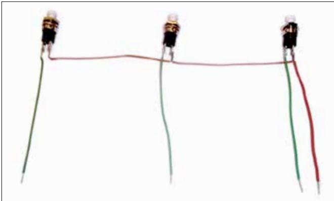
8. One lead of each pushbutton is wired to the others as a common connection.
