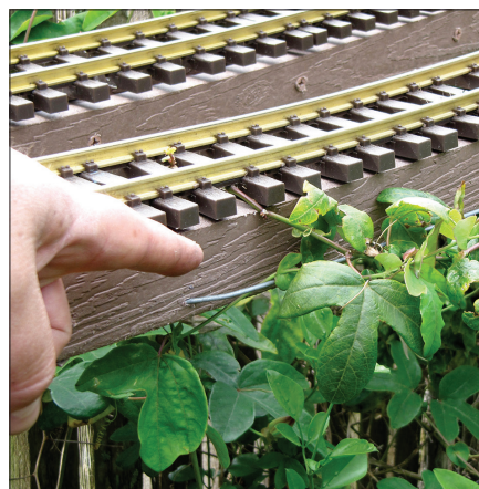
2. When you're passionate about running trains in your family's beautiful gardens, it helps to hide the mechanics of the benchwork. Steve shows how to make trackwork disappear amid passionflower vines.
