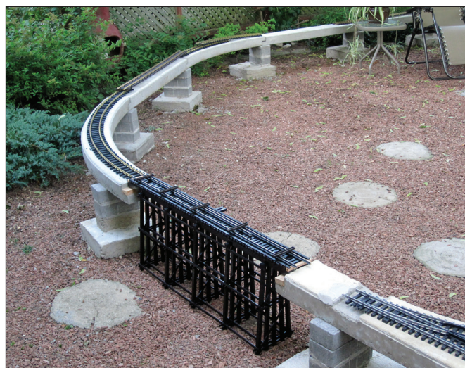
13. The finished system provides a firm and attractive roadbed.
