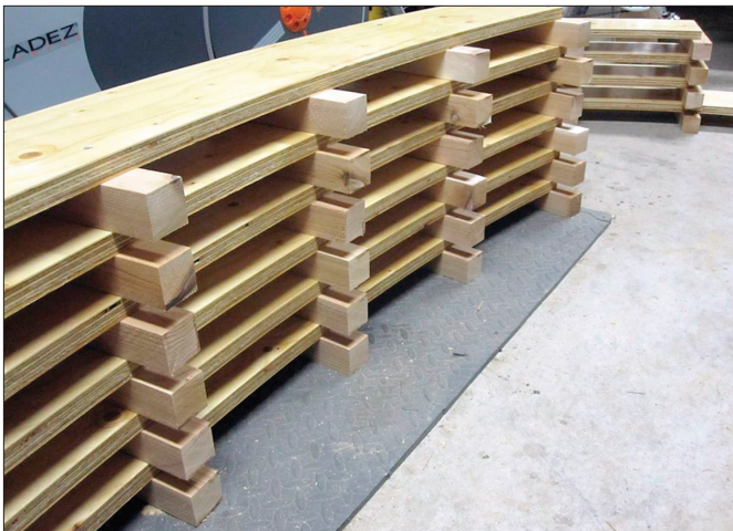
6. Wooden feet have been added to the bases.
