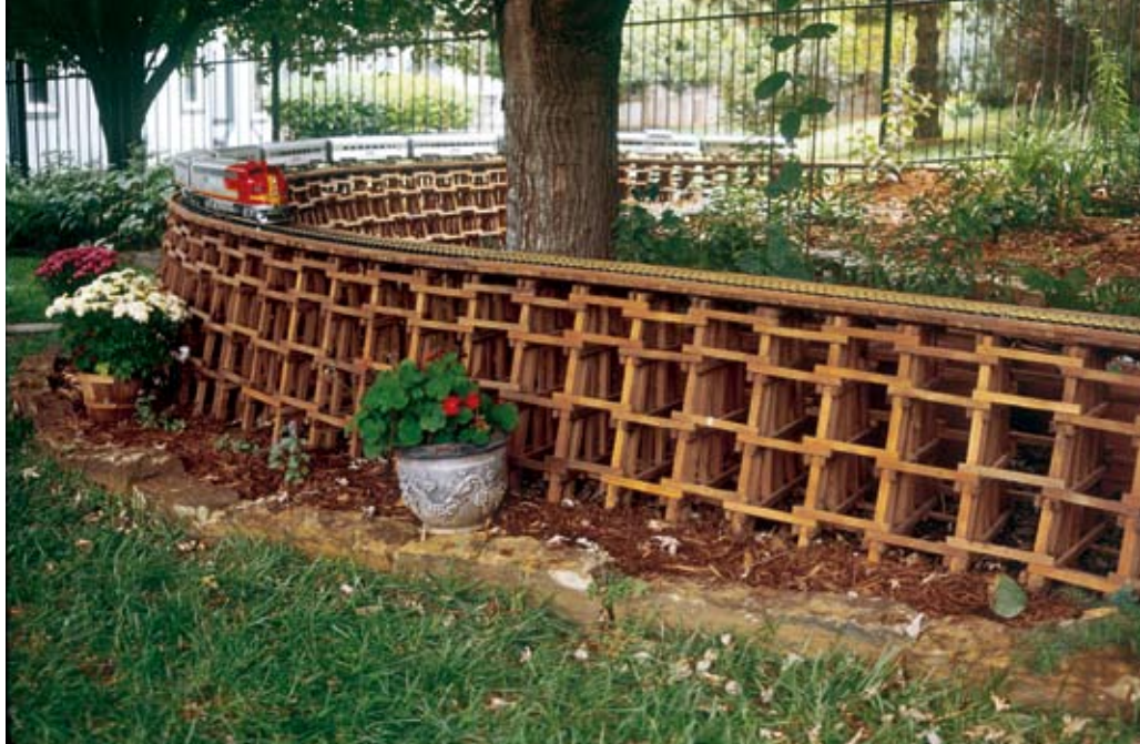
3. The 40' trestle keeps the L&R Railroad level as it traverses sloping land. The structure was built in sections, upside down on a workbench. Sections were dropped into place, then fastened together to form a single structure. Potted mums and geraniums can be switched around or moved to add color where and when needed.
