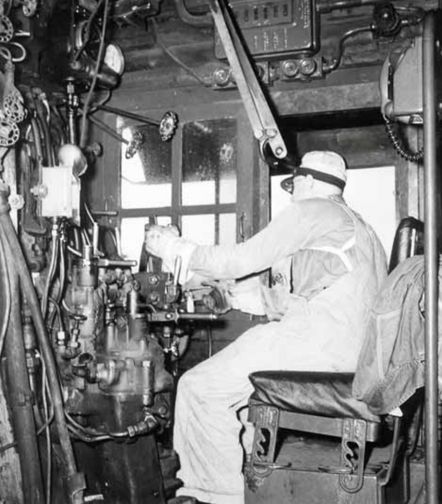
Two men and their machine: Engineer Ed App, his left hand on the reverse lever and right hand on the whistle valve, rolls 200 empty ore cars north from Proctor. Later, fireman John Shovein checks his fire before leaving Fraser with the loaded train.
