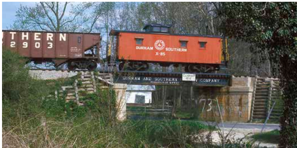
Fig. 1 I-beam bridge. This short and simple bridge on the Durham & Southern was made from standard steel I-beams set on concrete abutments.
