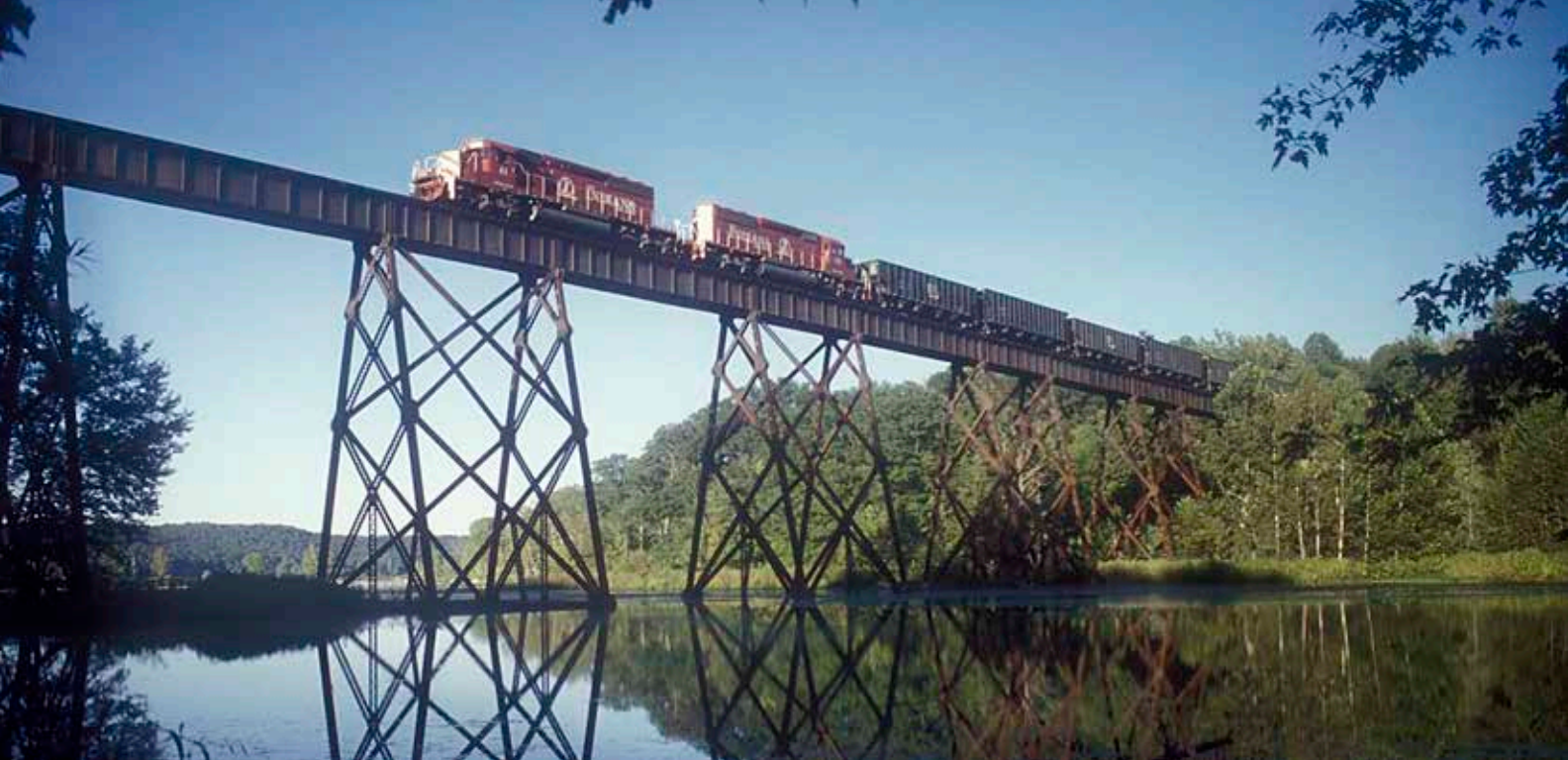
Fig. 8 Deck girder viaducts. Steel deck girder viaducts are made of fabricated I beams atop supporting towers. This bridge on the Indiana RR in southern Indiana has girders of identical depth regardless of their length. Some bridge designs use thinner girders for shorter spans.
