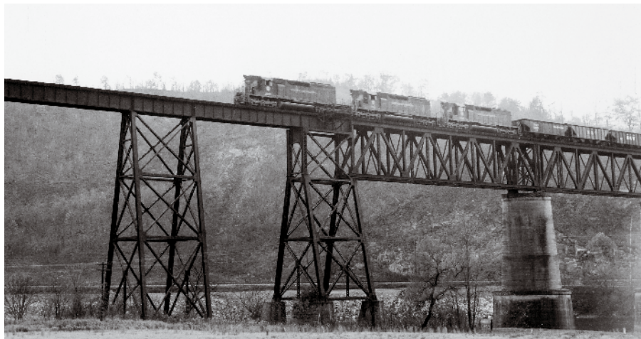
Fig. 8 Deck girder viaducts. Steel deck girder viaducts are made of fabricated I beams atop supporting towers. This bridge on the Indiana RR in southern Indiana has girders of identical depth regardless of their length. Some bridge designs use thinner girders for shorter spans.
