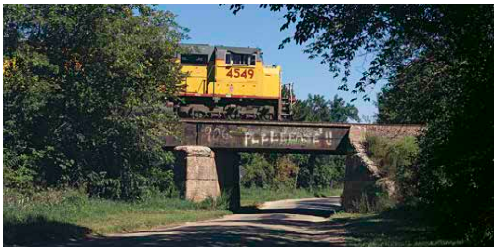
Fig. 2 Deck plate girder. This Chicago & North Western (Union Pacific) deck girder bridge was made from large I-beam shapes that were fabricated from plate steel. Bridges like this typically span 30- to 50-foot gaps. Carl Swanson photo
