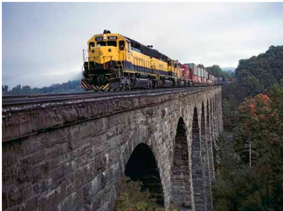
Fig. 6 Stone-arch viaduct. The Erie RR's massive Starrucca Viaduct in Lanesboro, Pa., was built from locally quarried stone in 1848. The bridge remains in active service today, more than 150 years after its completion. Note the "batter" (slope) of each pier. Matthew Van Hattem photo
