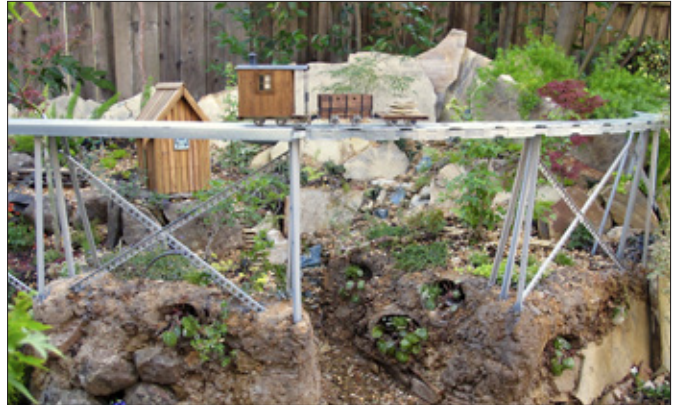
8. The author mixed one part peat, one part perlite, and one part Portland cement (by volume) with coloring to make hypertufa retaining walls, embedded with cantilevered metal trestle bents that model the 100-year old Alhambra trestle. The top steel roadbed (right), not yet finished, is made from 20-gauge Flex-C Trak. Pots sunk into the still-wet walls gave spaces for planting strawberry begonia and sweet alyssum. The gorge allows entry for maintenance.
