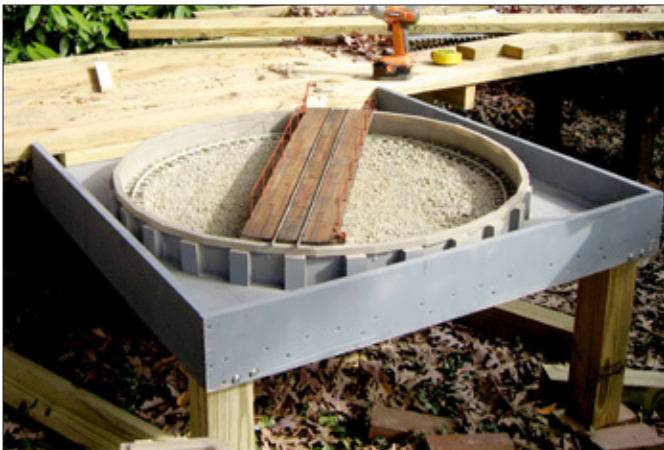
19. The turntable is installed.
