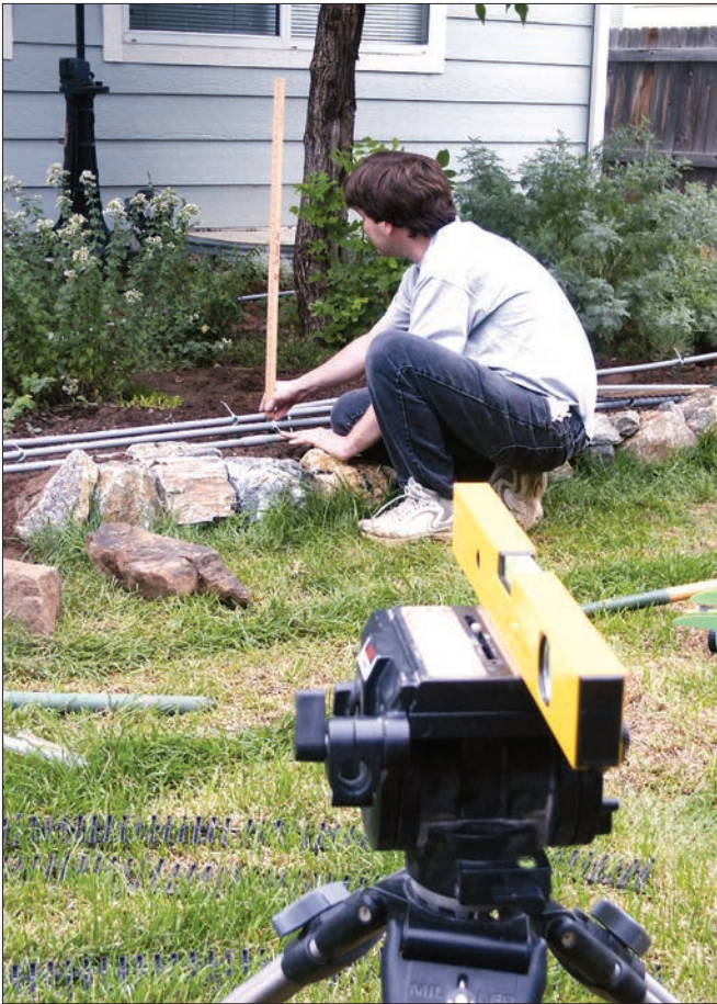
I use a laser level to accurately set the elevation of the subroadbed that will support the track on my Tuscarora Railroad. Ruth Strong
