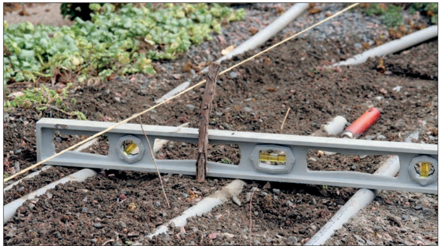
Sometimes, drastic measures must be taken to remedy a winter's worth of track movement. I used a string (stretched to be level across the length of the siding) and a 2' level to ensure that all three tracks of the yard at Neelyton are level. Once everything is leveled and the subroadbed tamped back in place, the track will be reattached to the PVC roadbed and new ballast spread over the track.
