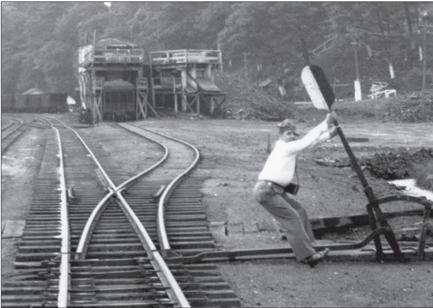
Stub switches were mostly gone from railroading by the early 1900s. This example is in Robertsdale, Penn., on the East Broad Top. A railfan identified only as Dave uses the harp switchstand to “bend the iron” and bend the rails to line up the switch. Kevin Strong collection
