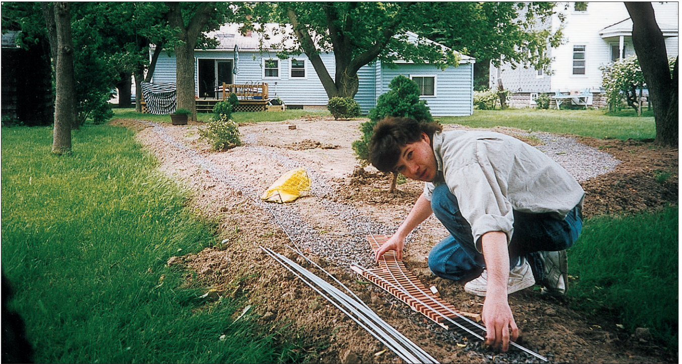
It's summer 1997, and I test-fit a new switch as I begin laying track on my former East Broad Top railroad in upstate New York. Forty yards of dirt were brought in to raise the railroad off the ground about 12" or so. Ruth Strong
