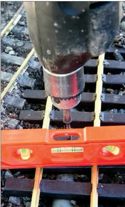
I attach my track to the PVC subroadbed with 1" deck screws. I leave the screws a bit loose and then check the level and adjust the ballast.
