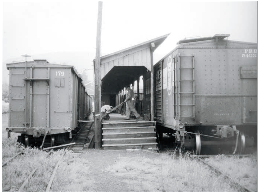
The size difference between standard and narrow gauge equipment becomes evident when seen side by side. This freight transfer shed at Mount Union on the East Broad Top is typical of many such facilities at places where two gauges came together. Incompatibilities in track gauge meant that freight had to be transferred from cars of one gauge to cars of the other. This was most often done by hand, which—even with cheap labor—meant a steady drain on profits. Narrow gauge is on the left and standard gauge on the right. The difference in track gauge is evident as well. Kevin Strong collection
