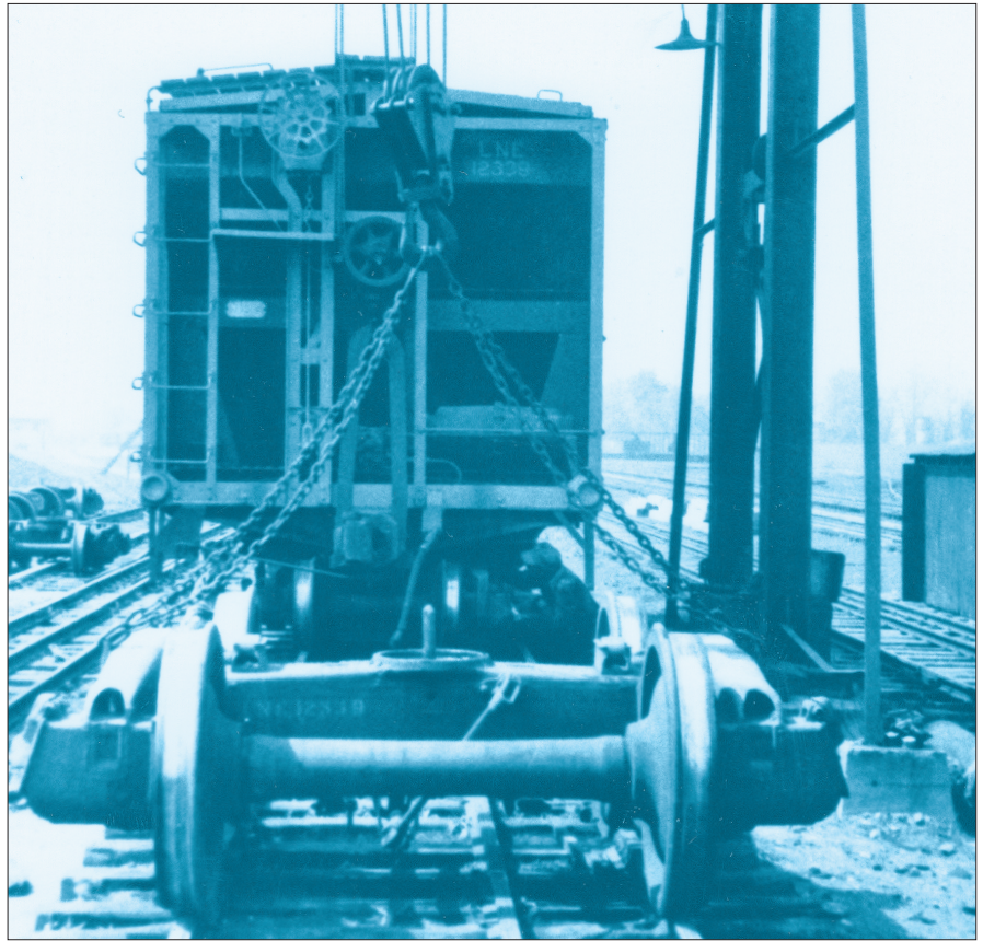
The East Broad Top Railroad remained viable into the 1950s, partly due to its practice of retracking standard gauge cars with narrow gauge trucks so standard gauge cars could operate on the EBT. This was accomplished by a large overhead crane. This cement hopper, being positioned on the narrow gauge trucks (standard gauge truck in the foreground) was one of many that moved over the EBT during the construction of the Pennsylvania Turnpike. Kevin Strong collection
