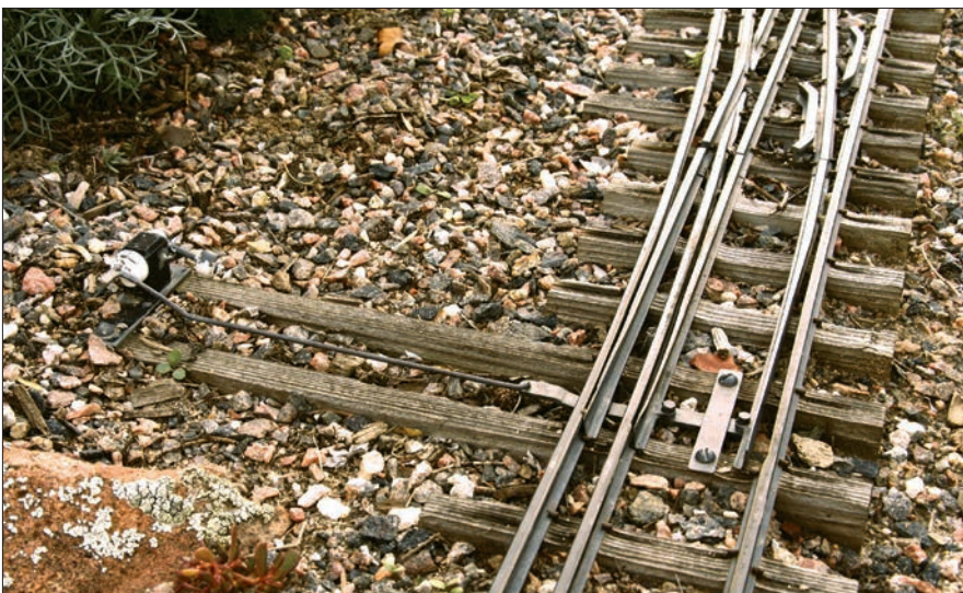
This rigid, ground-throw switch machine on the Ogden Botanical Railway is designed to hold the points against one rail or the other so that trains can pass smoothly through. The machine is rigidly attached to the throw bar to firmly set the points against the stock rails.
