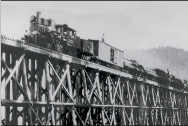
Logging railroads are popular in the garden. This photo shows the key elements: a logging locomotive, tall trestle, and loaded log cars. Photo courtesy Weyerhaeuser Historical Collection
