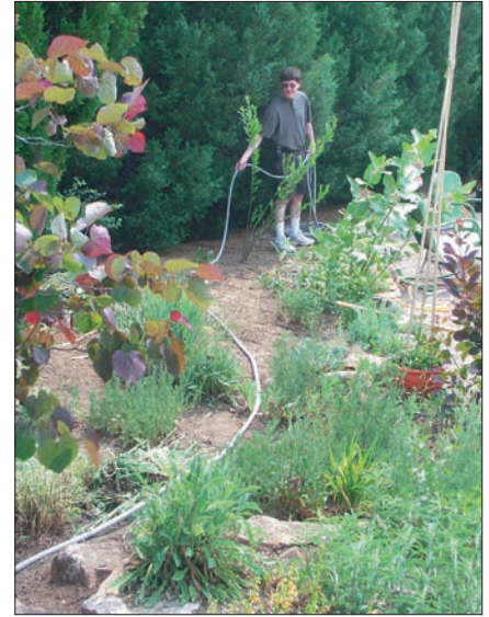
I use a garden hose to lay out the proposed track through an existing garden. Hoses give your eye a sense of where the track will go and how it will look. They also tend to form fairly smooth, even curves as you drape it around the landscape.
