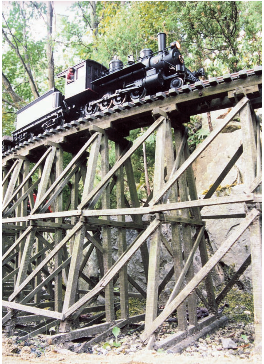
The engineer keeps a sharp eye out as he winds around the curved trestle on Jim Strong's Woodland Railway. A trestle is often the focal point of a garden railroad, and it's worth the time and effort to build one. They are not, however, indestructible as can be seen by the broken cross brace at the bottom.
