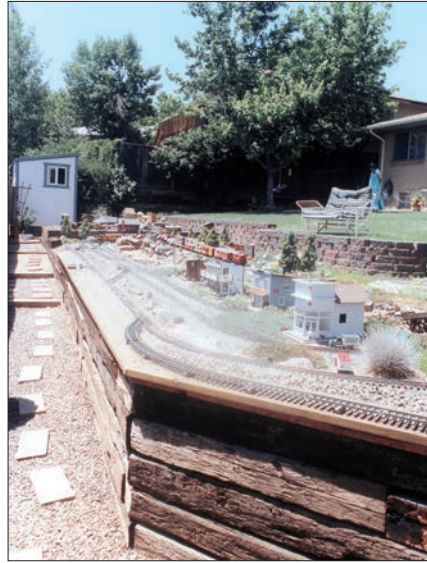
Railroad ties and landscaping blocks can be used to create a terraced garden area out of the sloping back edge of the yard. The terracing gives a formal boundary to the railway while elevating it to a workable height.
