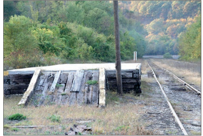
Simplicity in itself, this loading platform on the Mount Union Connecting Railroad waits for its next carload of freight in Mount Union, Penn. Nothing fancy, just old railroad tie cribbing filled with lots of concrete.
