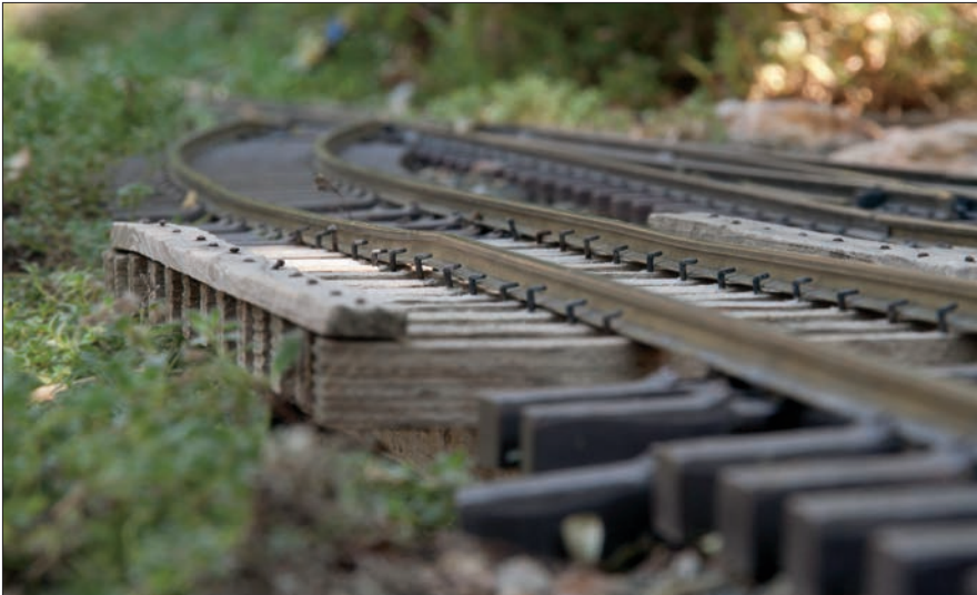
Kinks can be caused by many things, including someone stepping on the track or falling rocks and branches. Minor kinks can usually be massaged out of the track, while sharper ones warrant removal. This kink was caused when I tripped over the bridge. The most egregious bends of the kink were massaged out with pliers, but a slight vertical kink still remains. It's on a siding and has yet to cause a derailment, so it's low on the maintenance list.
