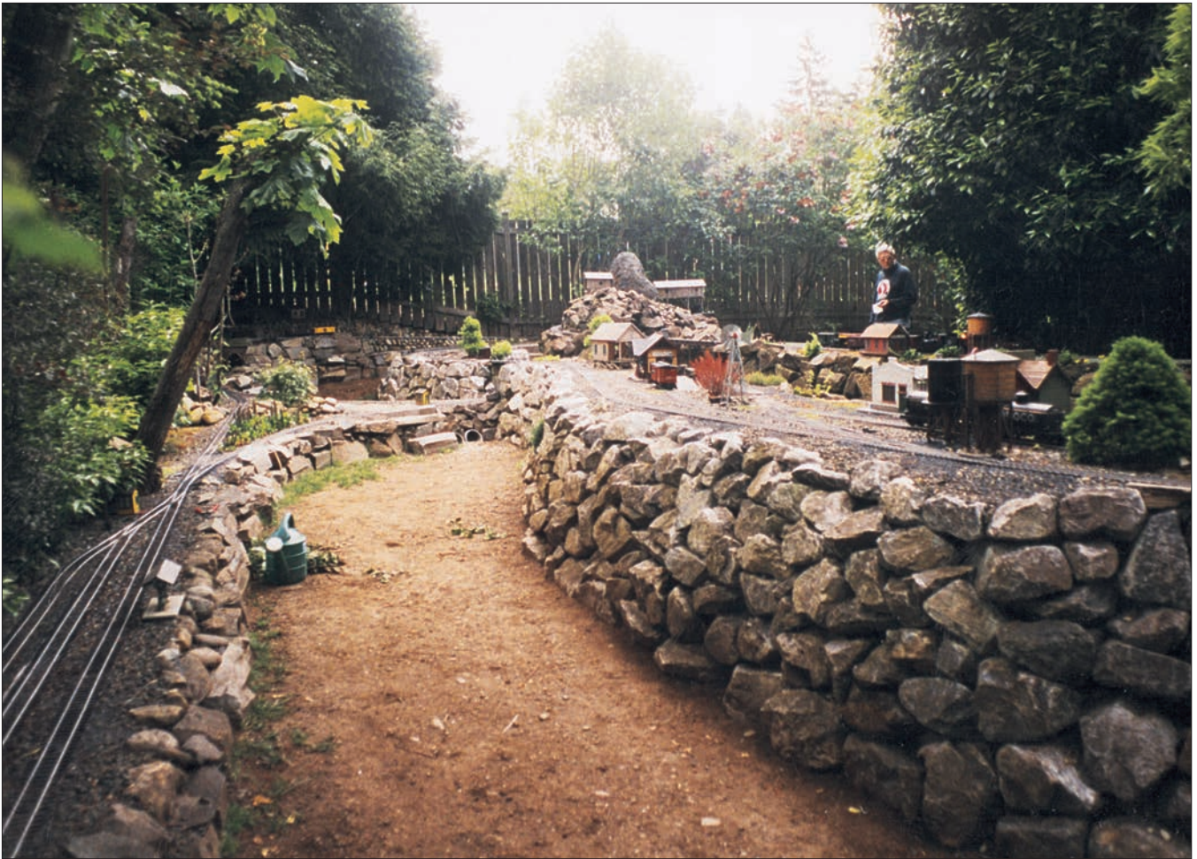
Retaining walls are often used to elevate a railroad to a more comfortable level. Here, Dave Goodson of Seattle has used large rocks to build up the peninsula in the middle of his railroad.
