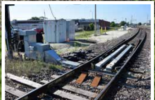
Full-size railroads use propane- or natural-gas-fired switch heaters (inset) to keep turnouts free of snow and ice in winter. Follow along as M.R. Snell explains how he modeled this common trackside detail in HO scale.
