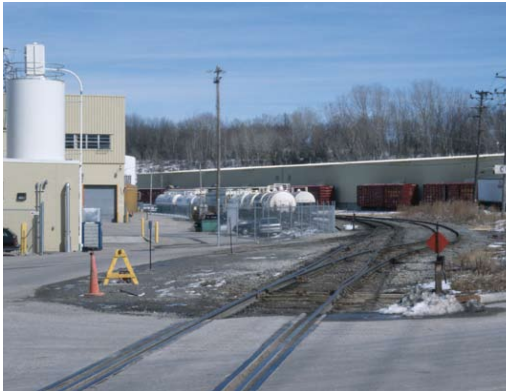
Paper mills are big, sprawling complexes of buildings. Here, a pair of spurs serve a chemical receiving area on one side of the main track, while boxcars are loaded with finished paper from the warehouse on the right. Photo by Jim Hediger
