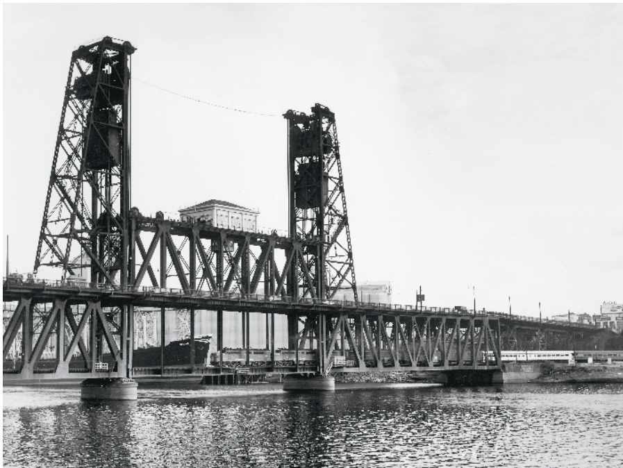
Portland Union Station is reached via the famed Steel Bridge over the Willamette River, which was engineered to allow the lower railroad span to be raised independent of the upper roadway. Henry R. Griffiths, Jr. photo
