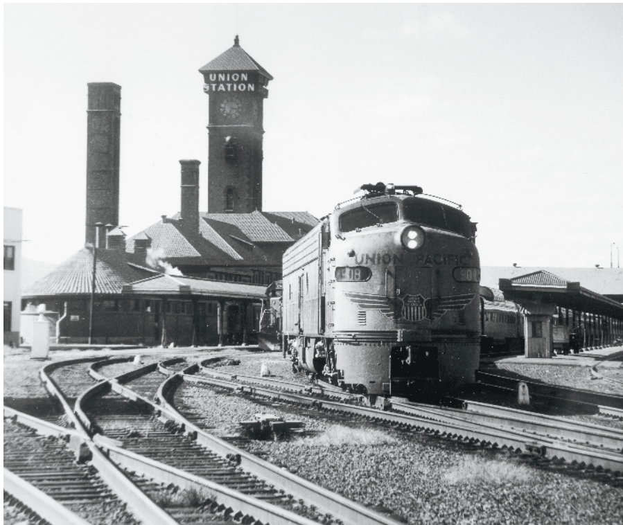
No model of Portland, Ore., is complete without the imposing brick Union Station. As shown here in September 1969, Union Pacific's eastward City of Portland is preparing to leave the station. Wayne Depperman photo
