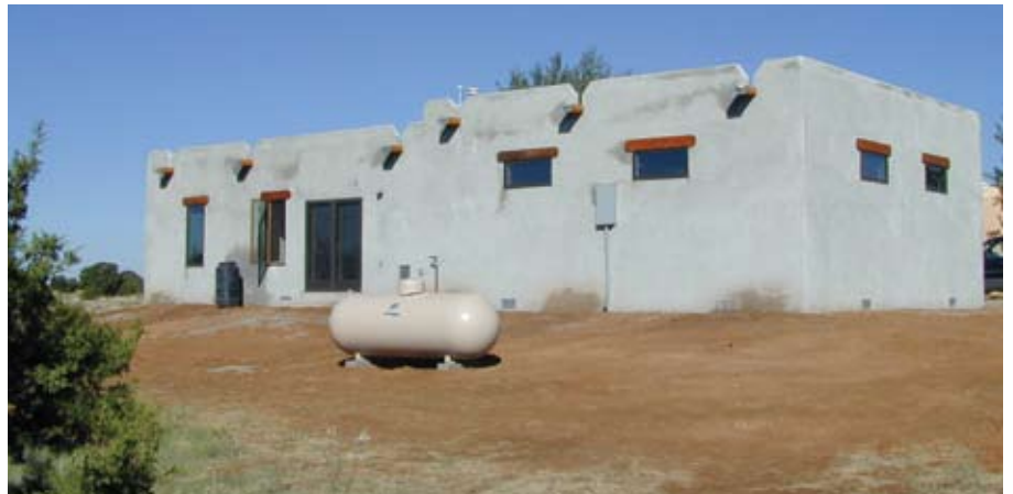
Bob Hayden had this adobe-style home-office and layout building factory-built to meet stringent local zoning codes and then transported the 28 x 60-foot building to his lot near Santa Fe, N.M. Bob Hayden photo
