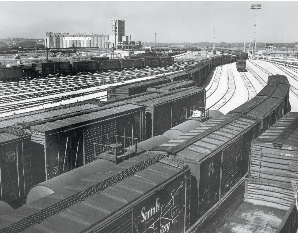
A '40s photo shows the east end of Elevator "A" with the six tracks that pass through loading and unloading sheds next to the tall work house. The west end of the Bowl Yard is visible at right. Santa Fe photo.
