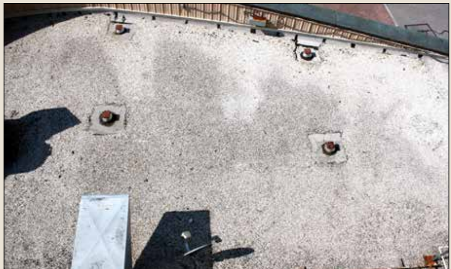
Gray pea gravel is another common surface treatment for modern flat roofs.
