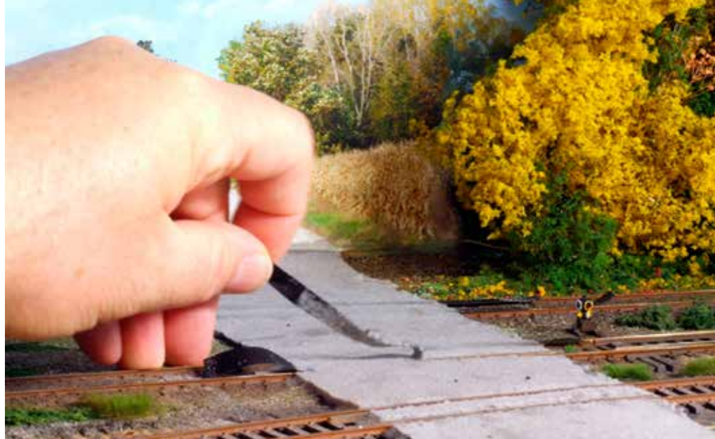
FIG. 3 LIFTING THE MASKS. After letting the diluted white glue securing the new road dry for about half an hour, Tom removes the tape on the edges of the road and the strips protecting the track's flangeways.
