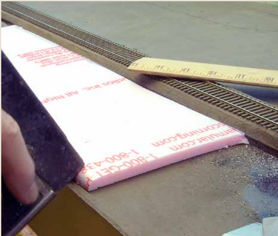
Fan-folded \frac{3}{8} " insulation board, sold at big-box or hardware stores, offered an easy fix. Tony cut strips to fit between the track and fascia or backdrop and stapled them in place using \frac{9}{16} " staples to fasten the foam along the outer edge.
