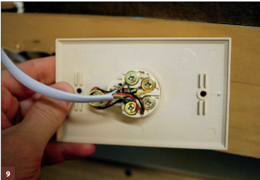
The cable is simply wired to the rear of the phone jack. On the NCE cab bus, the outer two wires are reserved for future use, so I was able to use a four-conductor jack.
