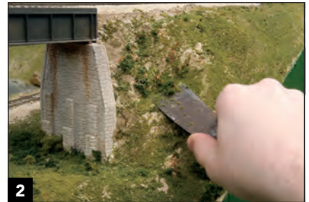
2 I used a putty knife to remove most of the old ground cover from the embankment.
