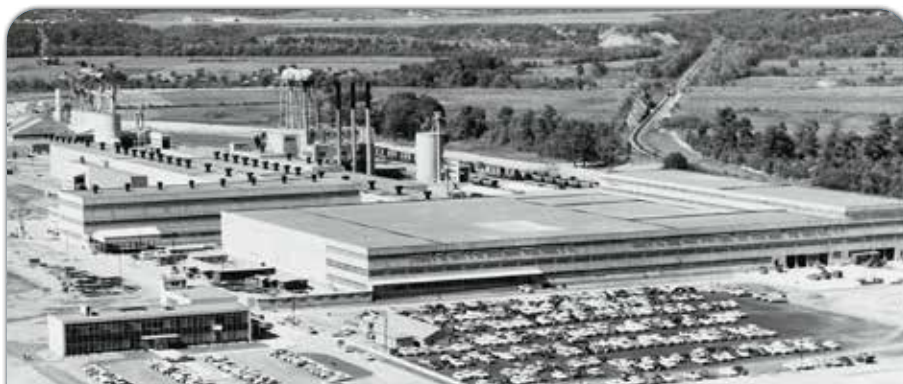
Pittsburgh Plate Glass Cumberland Works No. 7 produced glass in Cumberland, Md., from 1953 to 1981. For a time it was the only plant in the country with both a conventional rolled glass and float glass line. Photo courtesy of PPG
